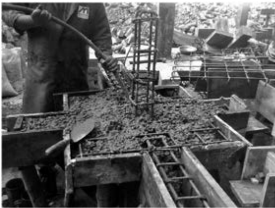
Fig 7. Concrete Casting of the Models
