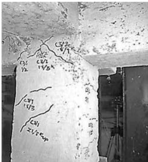
Fig 29. Joint Failure of Model 2
