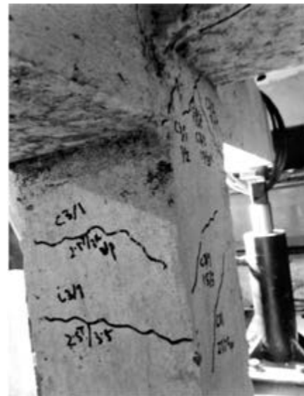
Fig 23. Column Failure, Model 2
