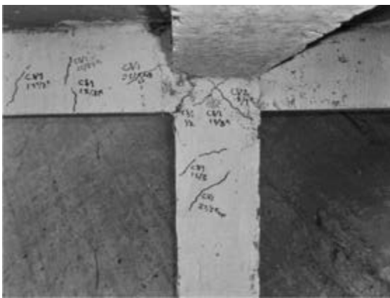
Fig 16. Model 2 Beam Cracks
