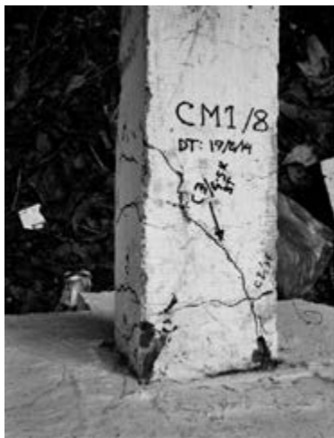
Fig 21. Upper Column Failure, Model 1
