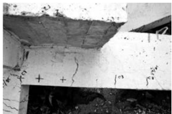
Fig 15. Model 1 Beam Cracks after Loading
