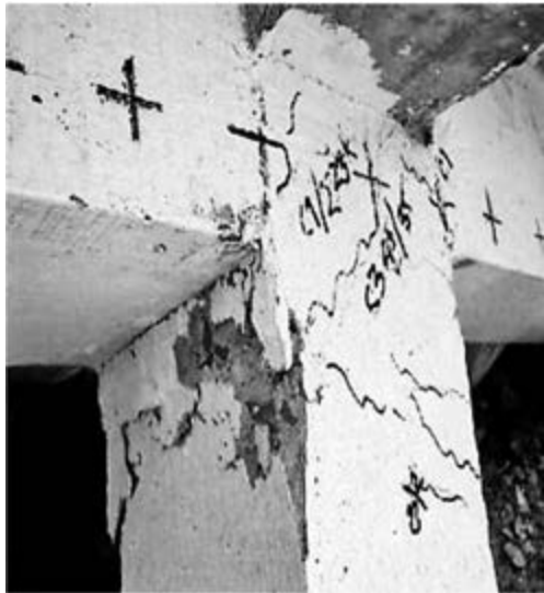
Fig 28. Joint Failure of Model 1
